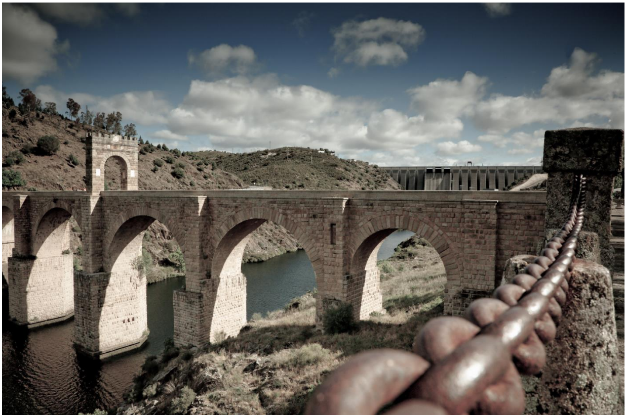
Alcántara Bridge, located near the intersection of the borders of the three regions Alentejo, Centro and Extremadura (Photo: Abraham Figuerido)
